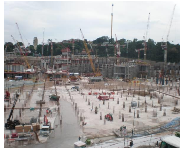
FOUNDATION WORKS AT CENTRAL ZONE, RESORTS WORLD AT SENTOSA
