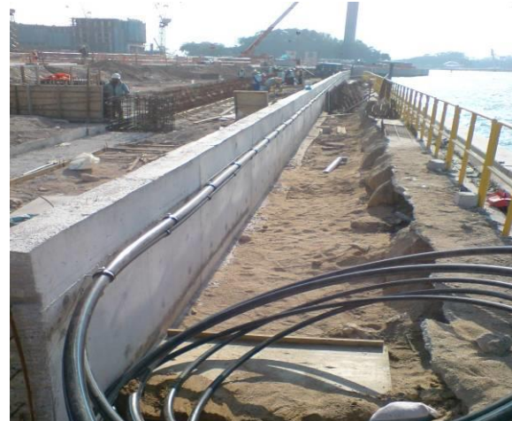
IRRIGATION MAINLINE & DECODER CABLE INSTALLATION
