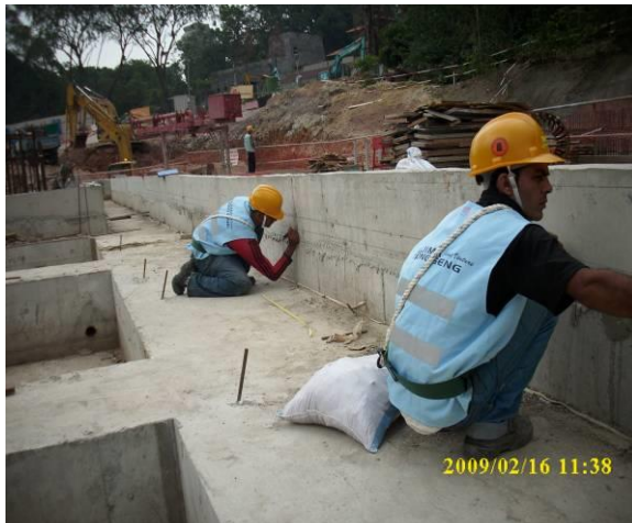
IRRIGATION MAINLINE & DECODER CABLE ALIGNMENT MARKING
