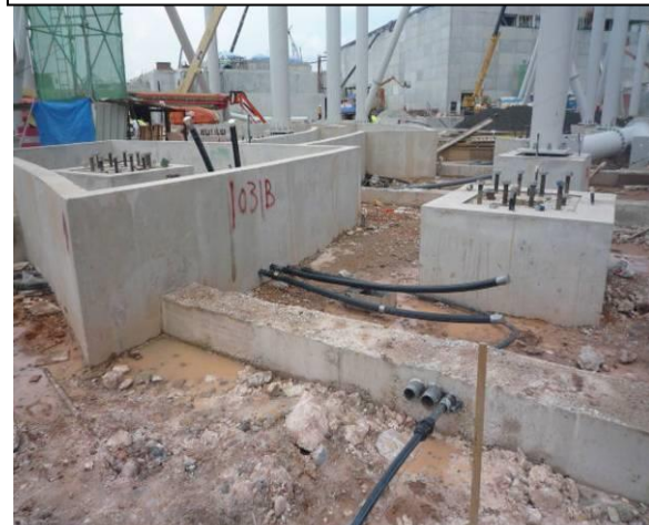
IRRIGATION SUBMAIN AND LATERAL CAST-IN PIPE
