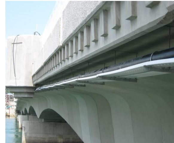
PIPE SUPPORT & TRAY INSTALLTATION AT SENTOSA BRIDGEWAY
