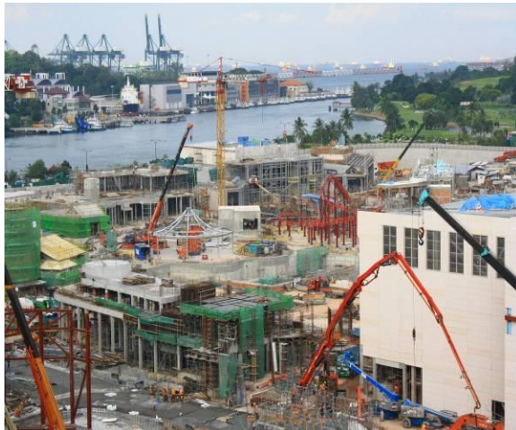
STRUCTURAL WORKS @ DREAMWORKS ZONE, UNIVERSAL STUDIO SINGAPORE
