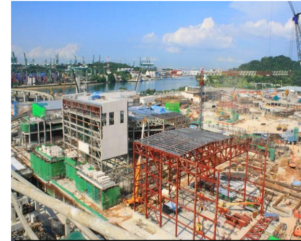
STRUCTURAL WORKS @ HOLLYWOOD & NEW YORK ZONE, UNIVERSAL STUDIO SINGAPORE
