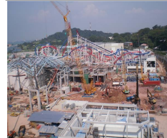
STRUCTURAL WORKS @ NEW YORK & SCI-FI ZONE, UNIVERSAL STUDIO SINGAPORE
