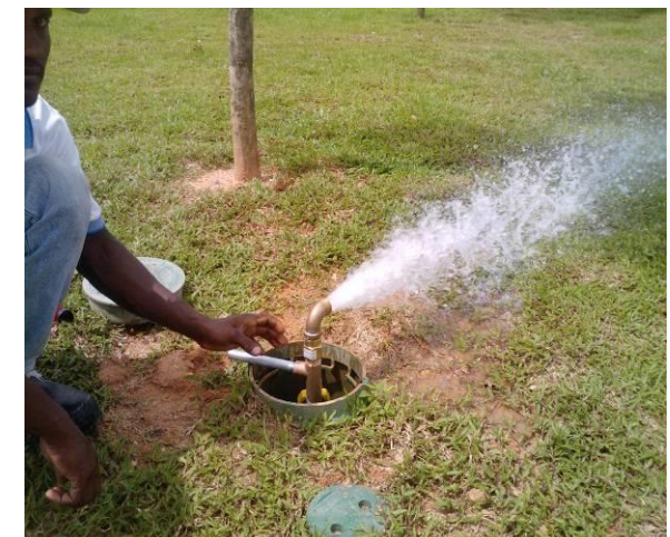
QUICK COUPLING VALVE AT PARK WIDE, RESORT WORLD AT SENTOSA
