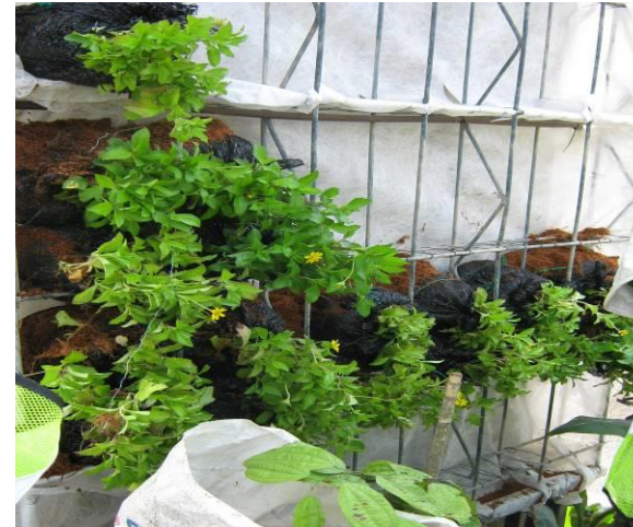
DRIP IRRIGATION AT GREEN WALL – SENTOSA MONORAIL PILLAR
