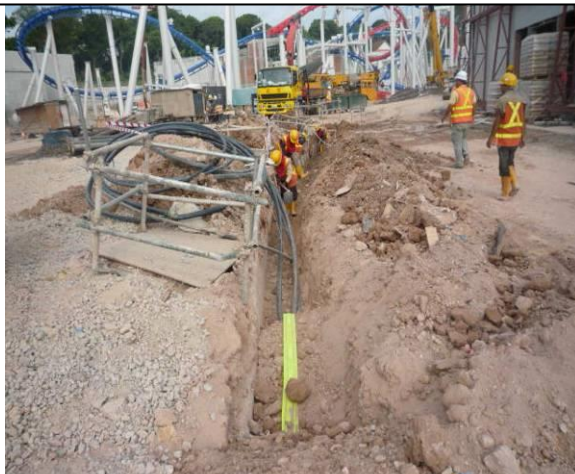
IRRIGATION MAINLINE & DECODER CABLE LAYING WORKS
