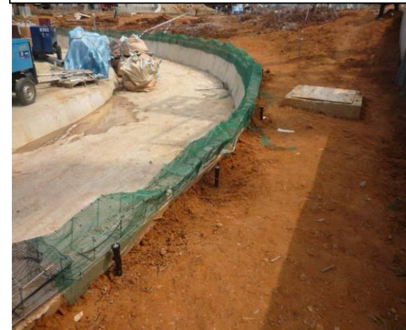
SPRINKLER INSTALLATION WORKS @ JURASSIC PARK ZONE, UNIVERSAL STUDIO SINGAPORE
