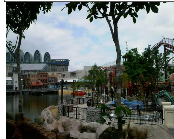
DRIPLINE LAYING WORKS @ DREAMWORKS ZONE, UNIVERSAL STUDIO SINGAPORE
