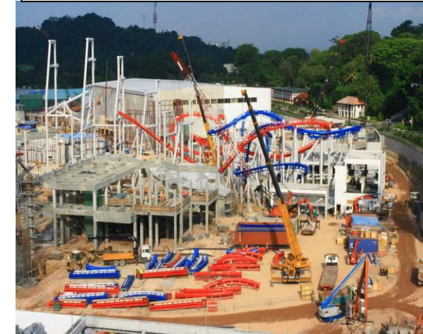
STRUCTURAL WORKS @ SCI-FI ZONE, UNIVERSAL STUDIO SINGAPORE
