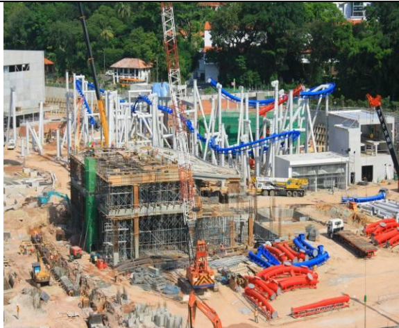
STRUCTURAL WORKS @ SCI-FI CITY & EGYPT ZONE, UNIVERSAL STUDIO SINGAPORE
