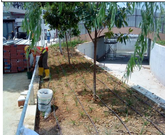
DRIPLINE LAYING @ WATERFRONT PLAZA, RESORTS WORLD SENTOSA
