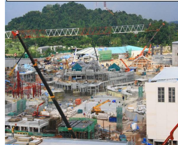
STRUCTURAL WORKS @ UNIVERSAL STUDIO SINGAPORE
