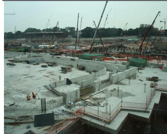
STRUCTURAL WORKS @ JURRASIC PARK & LOST WORLD ZONE, UNIVERSAL STUDIO SINGAPORE
