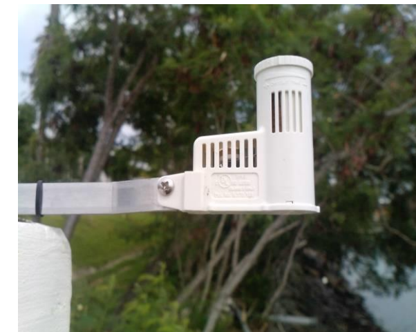
RAIN – CLICK / SENSOR AT SENTOSA IRRIGATION PUMPING STATION
