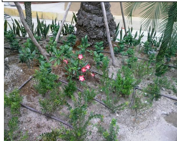
DRIPLINE LAYING WORKS @ EGYPT ZONE, UNIVERSAL STUDIO SINGAPORE
