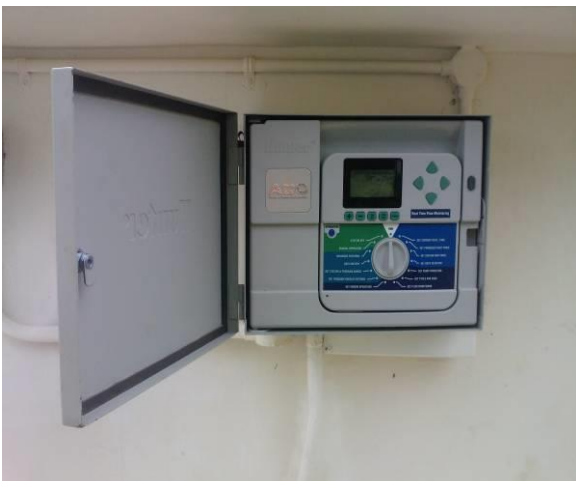
ACC CONTROLLER FOR GATEWAY AUTOMATIC IRRIGATION SYSTEM AT SENTOSA
