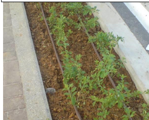
DRIPLINE LAYING WORKS @ CAUSEWAY, SENTOSA ENTRANCE
