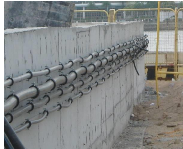
IRRIGATION MAINLINE & DECODER CABLE INSTALLATION
