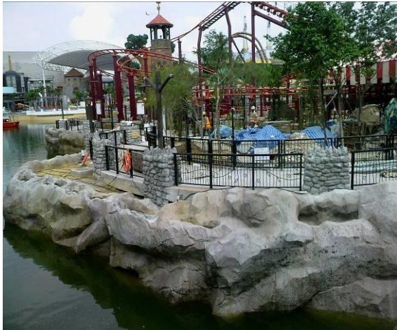
DRIPLINE LAYING WORKS @ FAR FAR AWAY ZONE, UNIVERSAL STUDIO SINGAPORE
