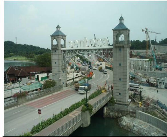
STRUCTURAL WORKS - SENTOSA ISLAND BRIDGEWAY ENTRANCE AT SINGAPORE
